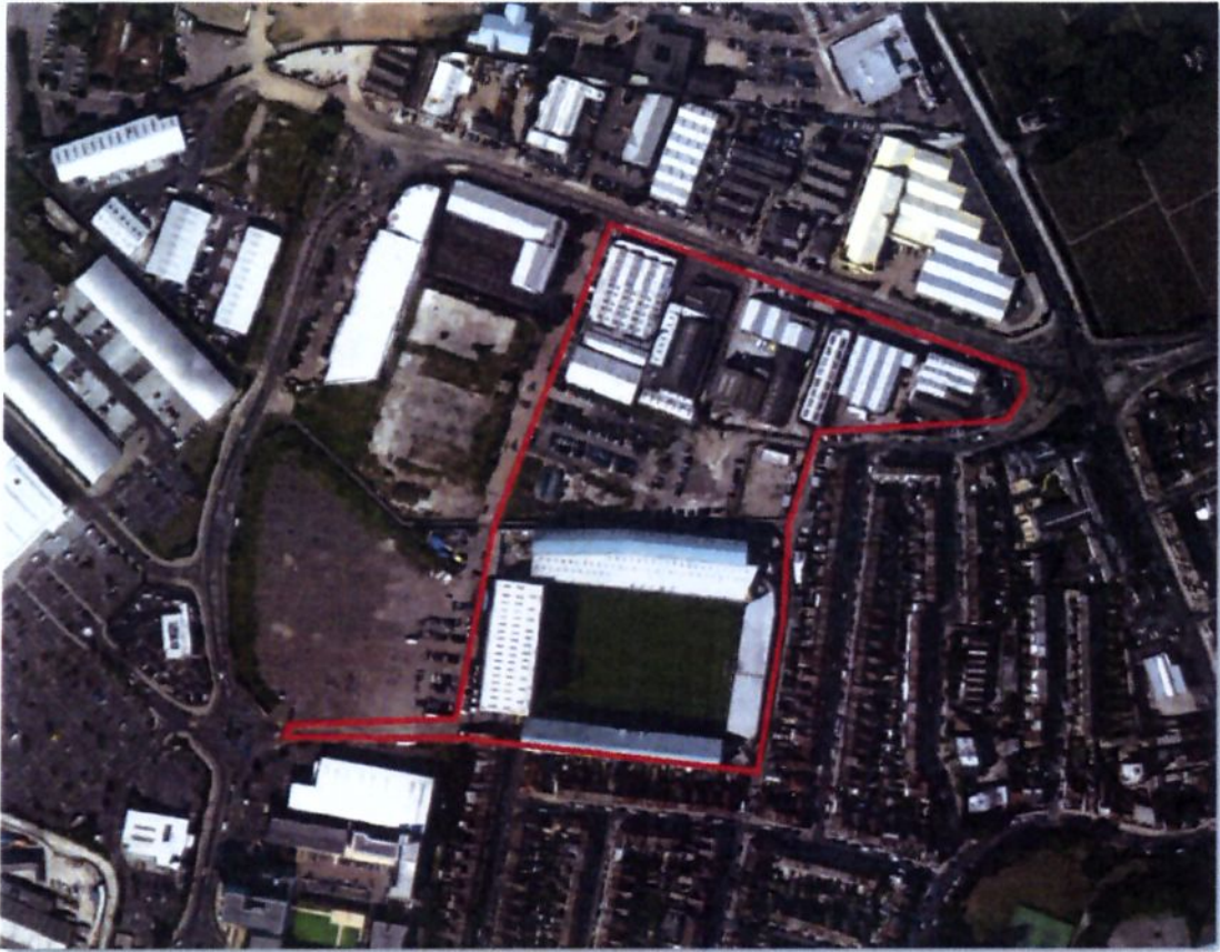
Figure 03: Aerial photograph of 'the site' (bordered red) [image obtained from Google Maps]
